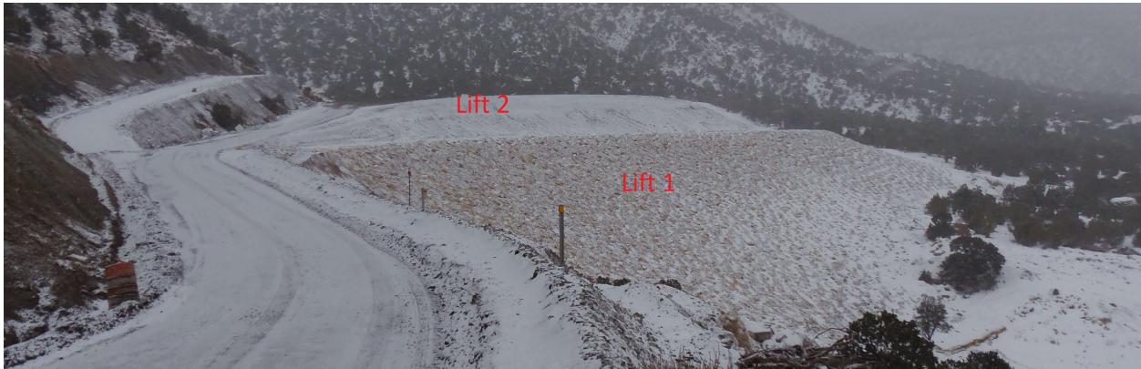
SCA#2 Ash Landfill – lower face looking easterly
