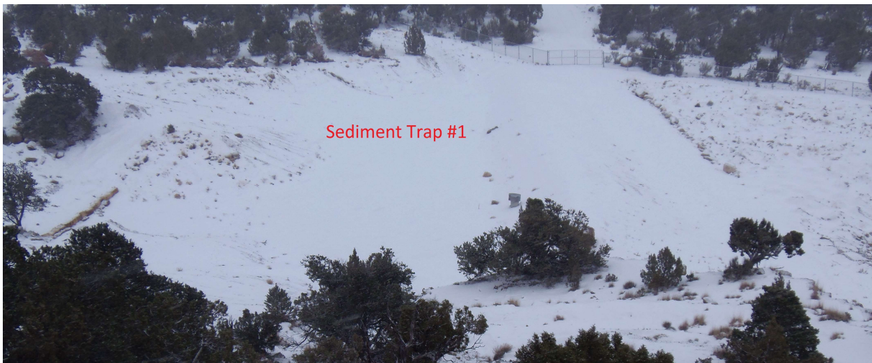
Sediment Trap #1, located immediately west of landfill – photo looking southerly
