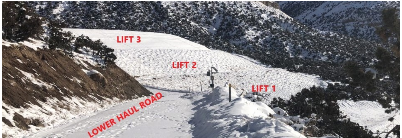
SCA#2 Ash Landfill –looking southeasterly
