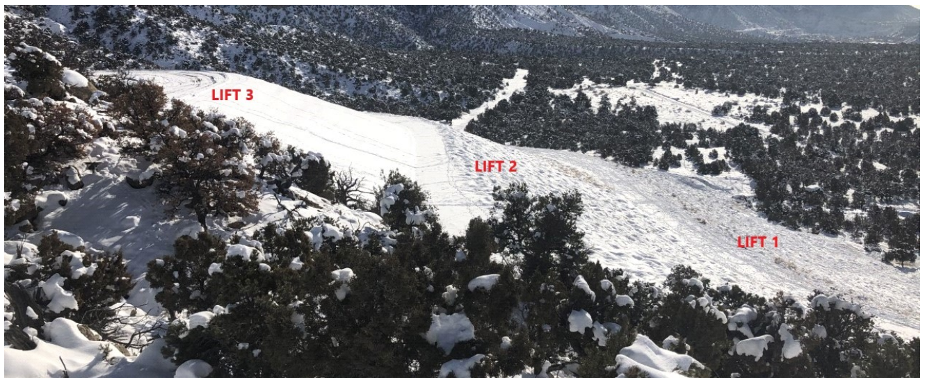
SCA#2 Ash Landfill – west face looking southerly Lift #1 and #2 covered and seeded. Lift #3 in process
