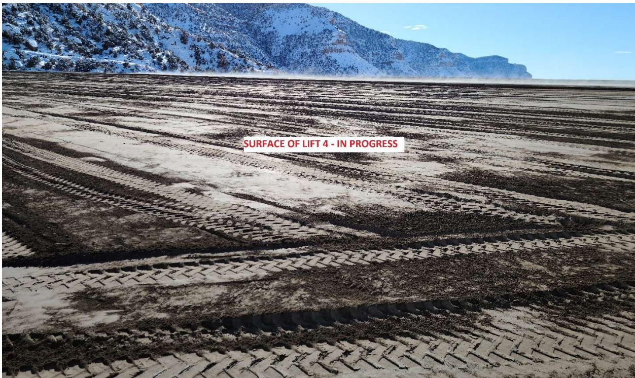
Surface of Lift #4 in progress – photo looking west - southwest Compaction appears satisfactory. Dust suppression appears satisfactory Surface slopes east towards the hill to prevent storm water run-on
