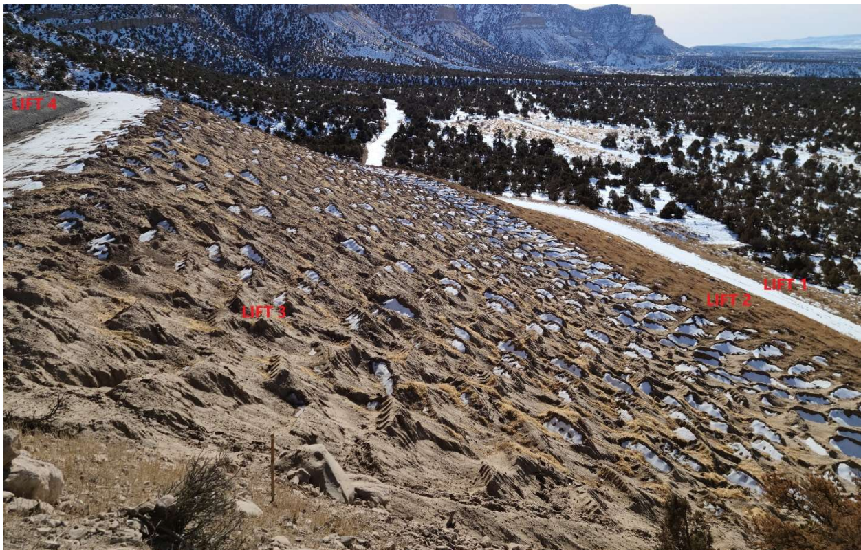
SCA#2 Ash Landfill – west face looking southerly Lift #1, #2 and #3 covered and seeded. Lift #4 in process
