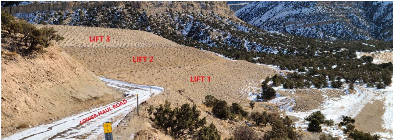
SCA#2 Ash Landfill –looking southeasterly
