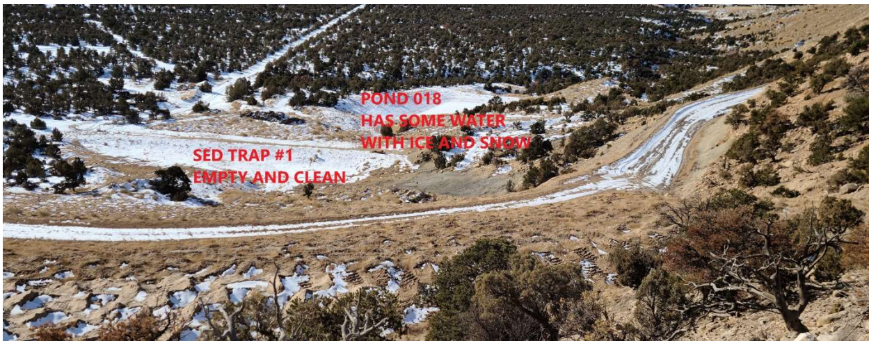
Sediment Pond 018, located west of Sed Trap #1 – photo looking westerly Pond has water with a surface ice layer and recent snow cover. No discharge in 2020 Sediment Trap #1 is empty and clean, water flows from trap to pond in normal open condition.
