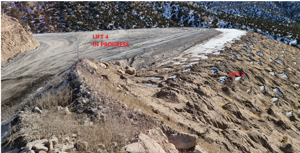
Surface of Lift #4 in process – photo looking south-southeast January 14, 2021
