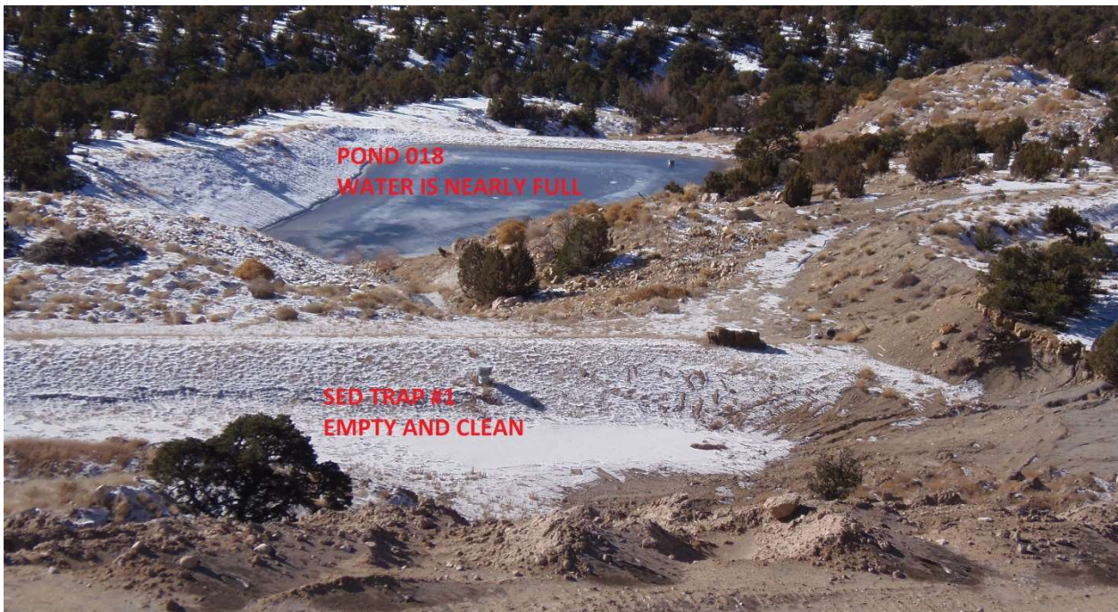
Sediment Pond 018, located west of Sed Trap #1 – photo looking westerly
