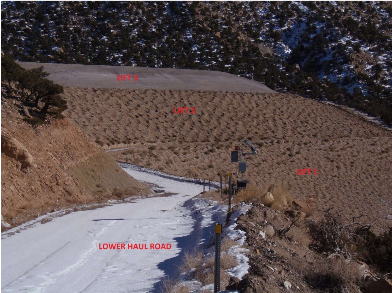
SCA#2 Ash Landfill –looking southeasterly
