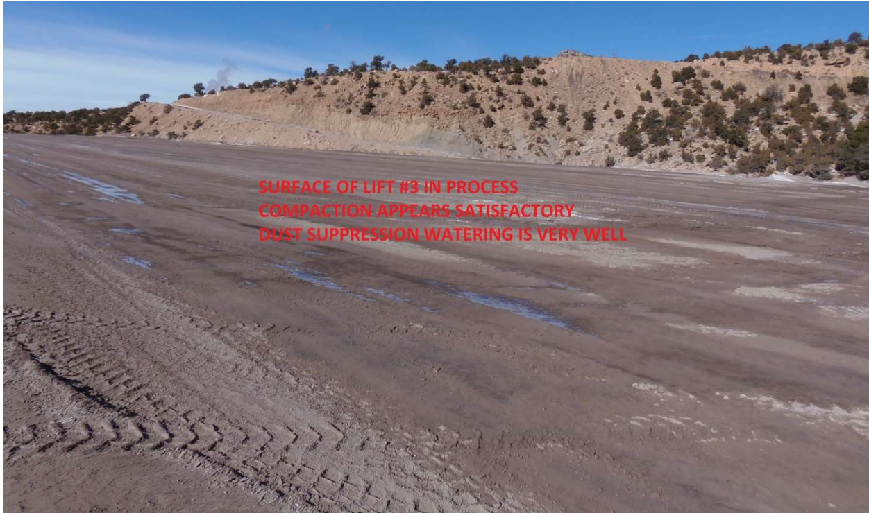
Surface of Lift #3 in process – photo looking northwesterly
