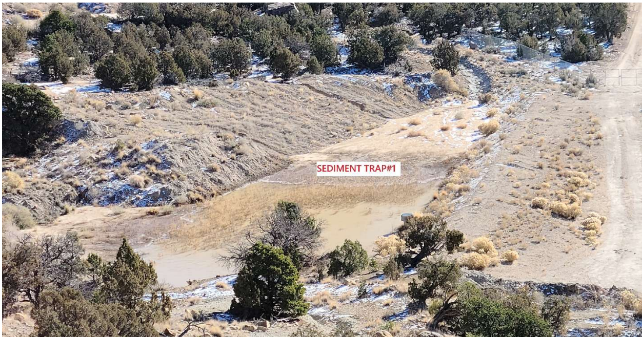
Sediment Trap #1 is has some water water flows from trap #1 to pond 018 in normal open condition
