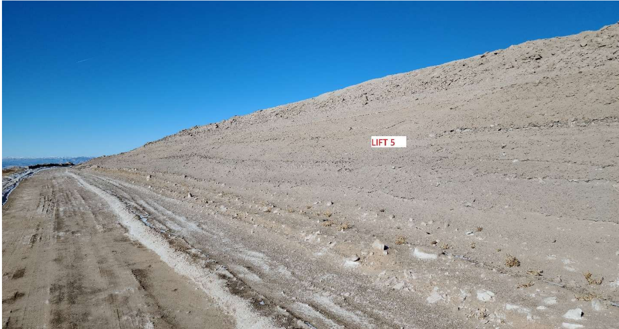
Lift #5 – in process – photo looking northwest
