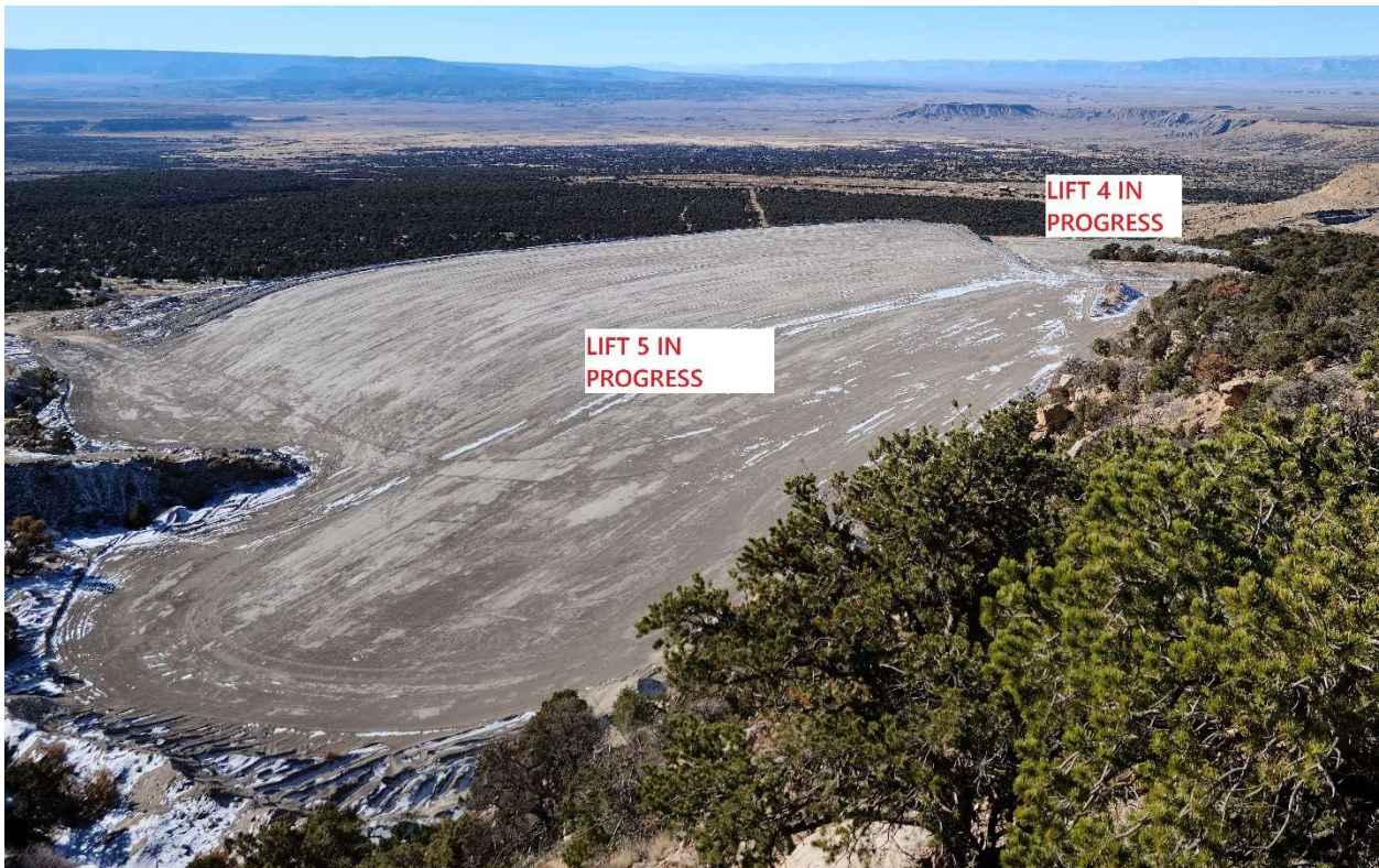
SCA#2 Ash Landfill – looking westerly Lift #5 in progress
